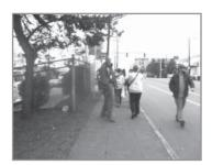
This narrow sidewalk does not accommodate the pedestrians that use it, especially before and after the adjacent middle school hours. The sidewalk does not have a planter strip to buffer the pedestrians from traffic. In this photo, a pedestrian chooses to walk in the street to avoid other pedestrians
